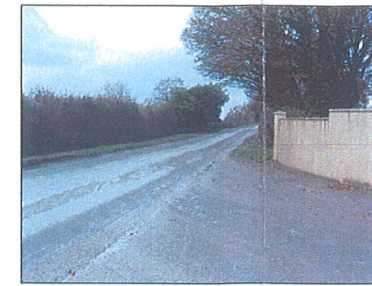
PHOTO 1 - VIEW TO RIGHT FROM EXISTING ACCESS
